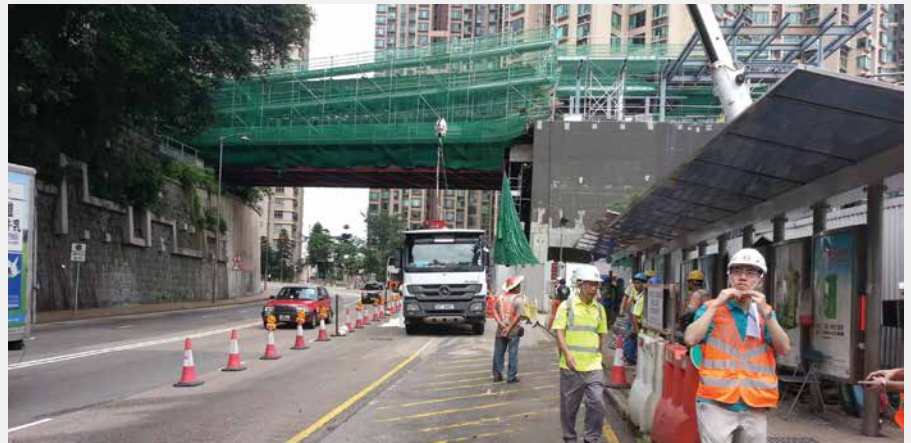
Two prefabricated working platforms were lifted and set up over a busy traffic road at Pok Fu Lam.
