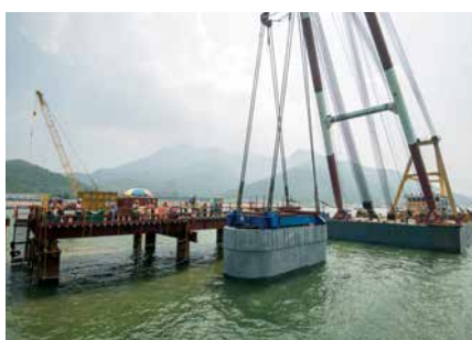
A 500-tonne-capacity marine barge lifting precast pile cap shell.
